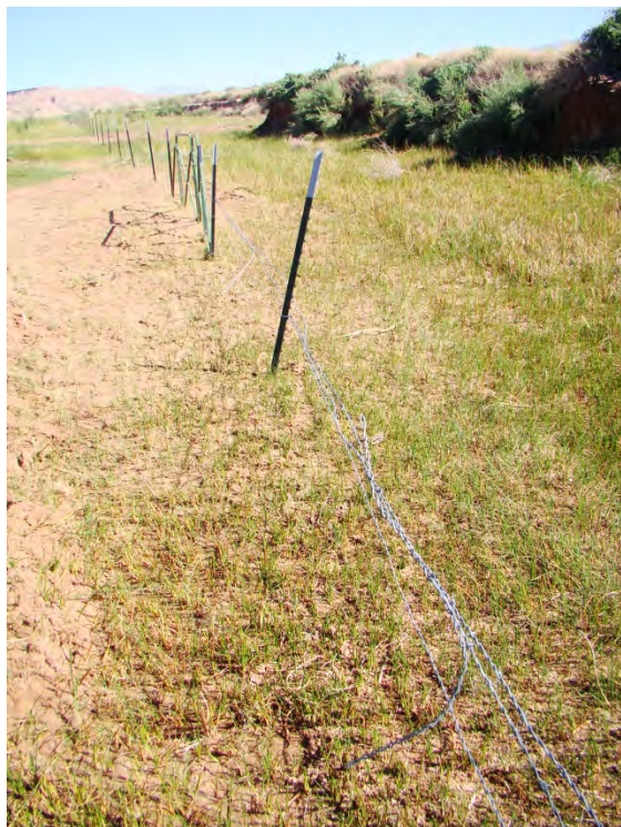
Location where cattle took down the fence and entered the site
