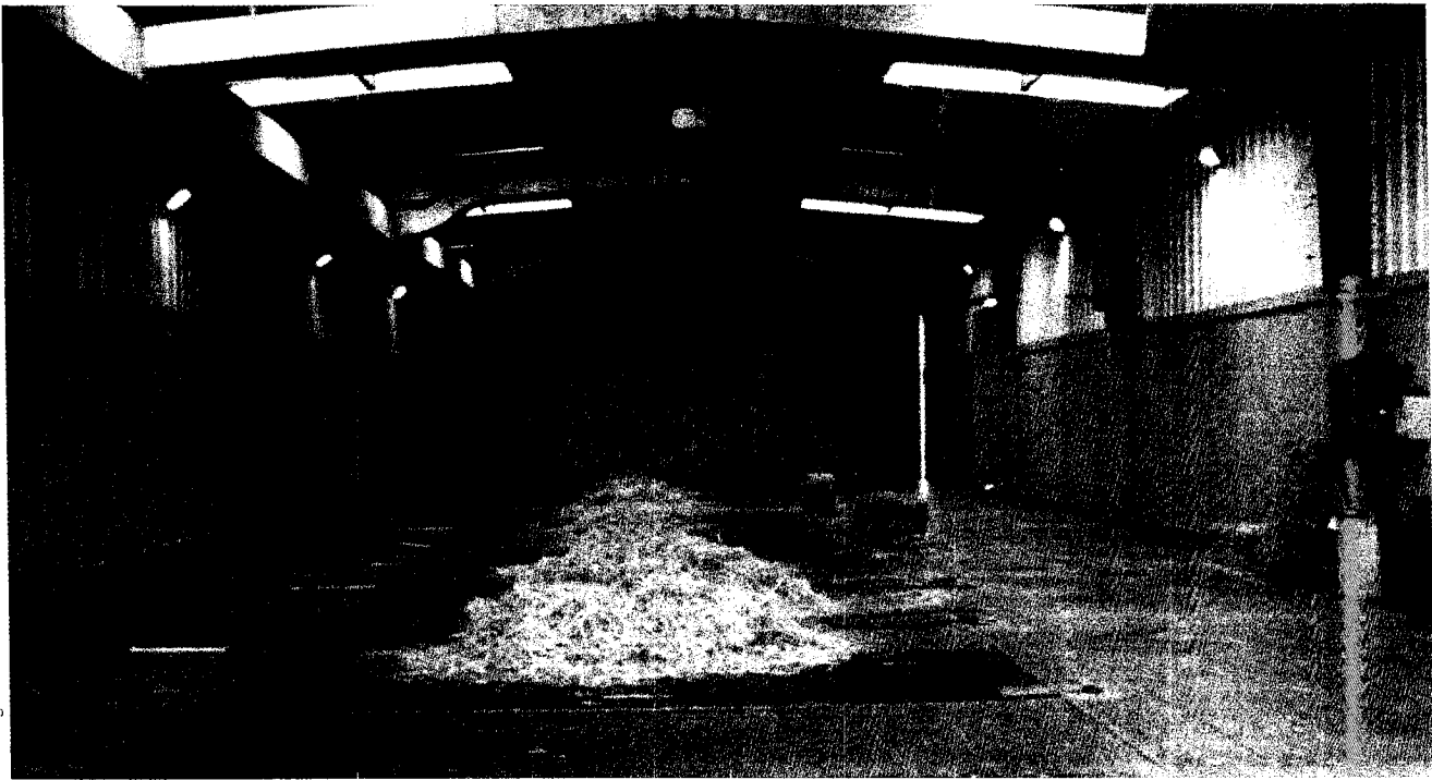
Concrete can act as a heat sink, chilling elephants that lie directly on it. Rubber mats and/or bedding of straw or sawdust can be used to keep the elephants more comfortable.
