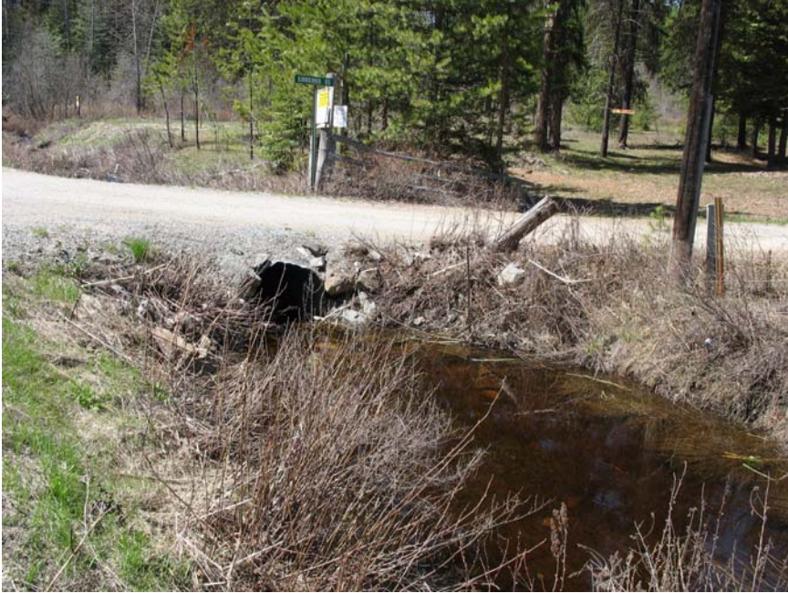
Photograph 9 - View of outlet channel on north side of Kalispell Bay Road flowing west toward Kalispell Creek
