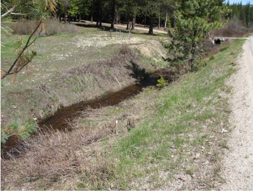
Photograph 11 - View of outlet channel on north side of Kalispell Bay Road flowing west toward Kalispell Creek
