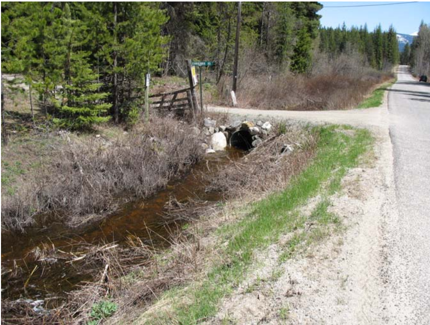
Photograph 10 - View of outlet channel on north side of Kalispell Bay Road flowing west toward Kalispell Creek
