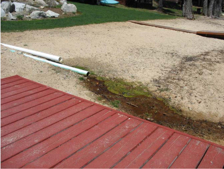
Photograph 19 - Drainage pipes at shoreline of Priest Lake south of Sackett property
