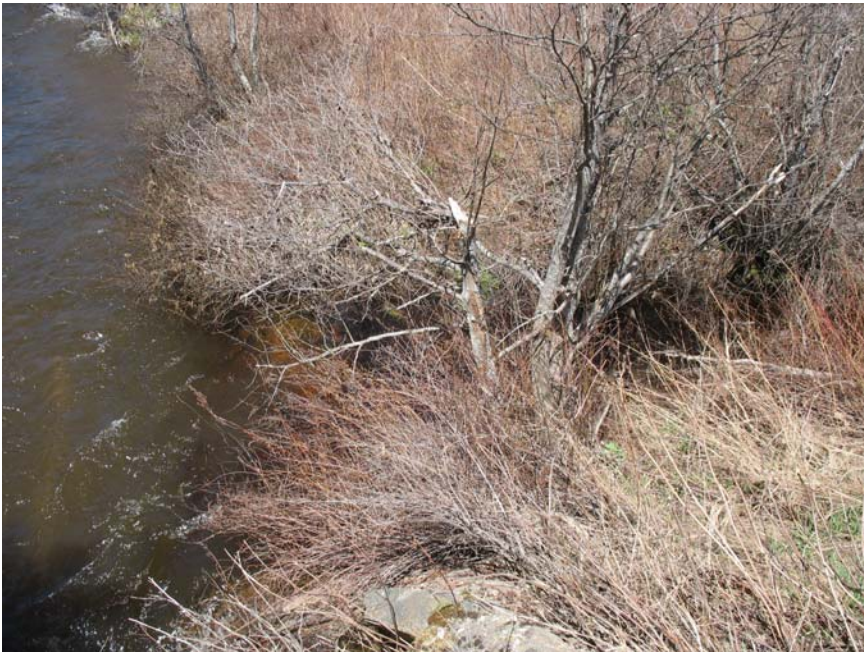
Photograph 12 - Mouth of outlet channel at Kalispell Creek on north side of Kalispell Bay Road
