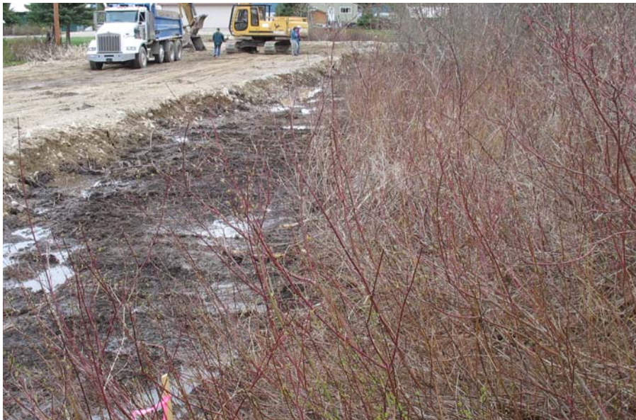
14) Red-twigged vegetation in the foreground is red osier dogwood. The stake delineates the northwest lot corner.
