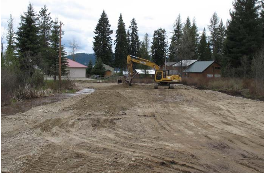
1) Excavator filling excavated wetland site, Mike and Chantell Sackett's lot.
