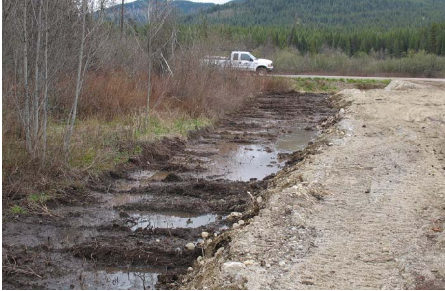
3) Same excavated area in photo 2, photographed from the south with the neighboring property of intact wetlands on the left, fill on the right.
