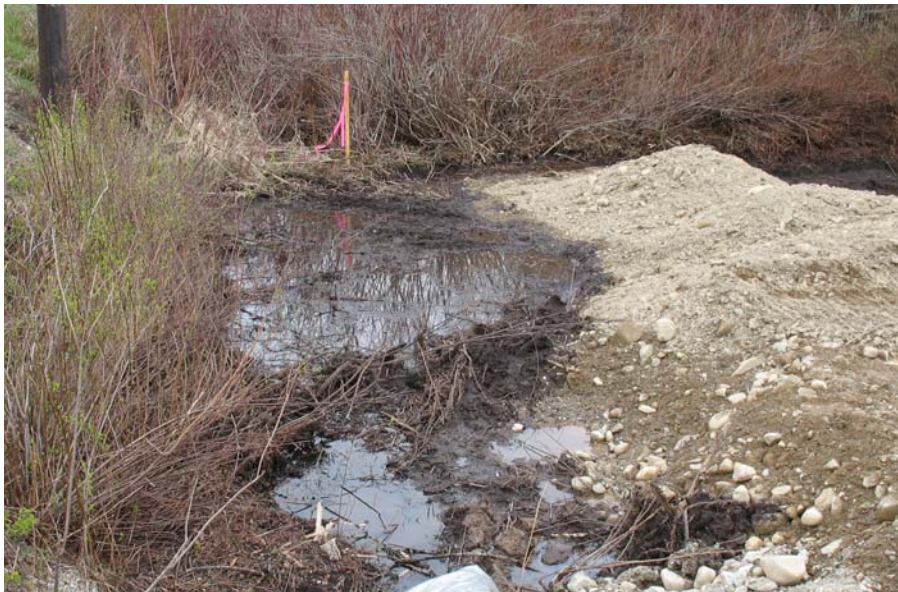
8) Culvert placed at entrance to the lot.
