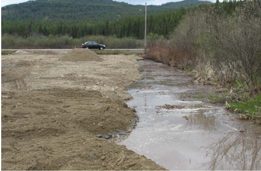
7) East side of the lot showing a strip of excavated ground that was being filled when we arrived.
