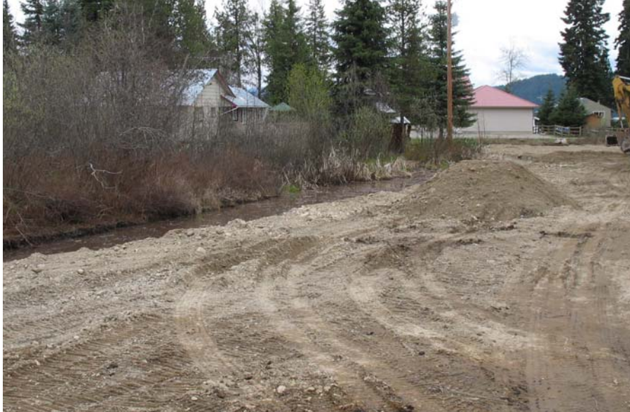
9) East side of lot showing the excavated strip that was being filled when we arrived, and backyard of the neighbors to the east.
