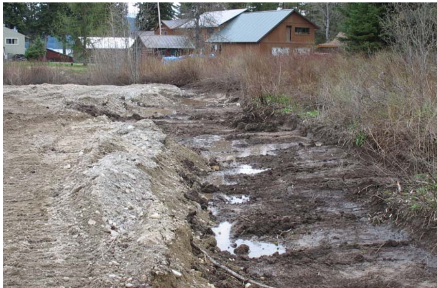
2) West side of lot showing a strip of excavated ground on the right abutting the neighboring property of intact wetlands; fill shown on the left.
