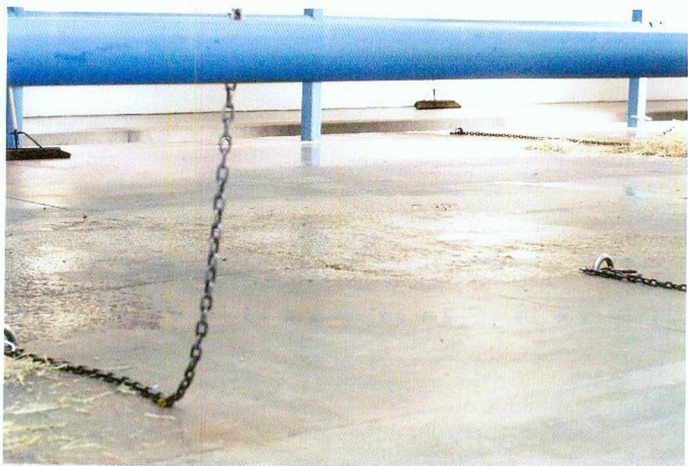
Fig. 51- PL 15568 Concrete floor surface of barn with elephants' foot wear patterns.
